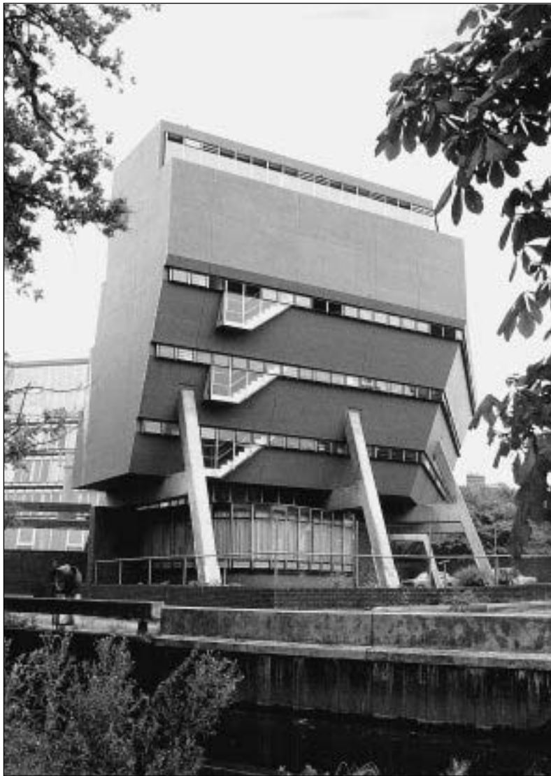
Fig. 5.17 Florey Building, Oxford, UK, 1971; James Stirling, architect. The Florey Building, with its crescent-shaped plan, complex cross-section and glazed wall, illustrates how the geometric freedom made possible by a continuous frame of in situ concrete can be exploited. (Photo: P. Macdonald)
