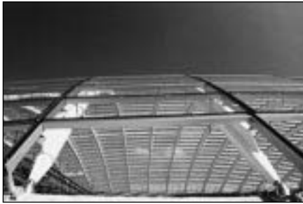
Fig. 7.53 National Botanical Garden of Wales, 1999; Foster and Partners, architects, Anthony Hunt Associates, structural engineers. This innovative single-layer dome is a toroidal form executed in one-way-spanning tubular steel arches, of varying span, with orthogonal linking elements. Built form of this complexity in steelwork was not possible before the age of computer-aided design.
