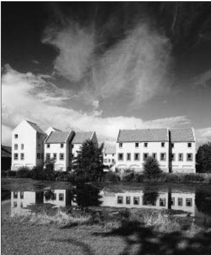
Fig. 1.14 Local authority housing, Haddington, Scotland, 1974; J. A. W. Grant, architects. These buildings have loadbearing masonry walls and timber floor and roof structures. (Photo: Alastair Hunter)
