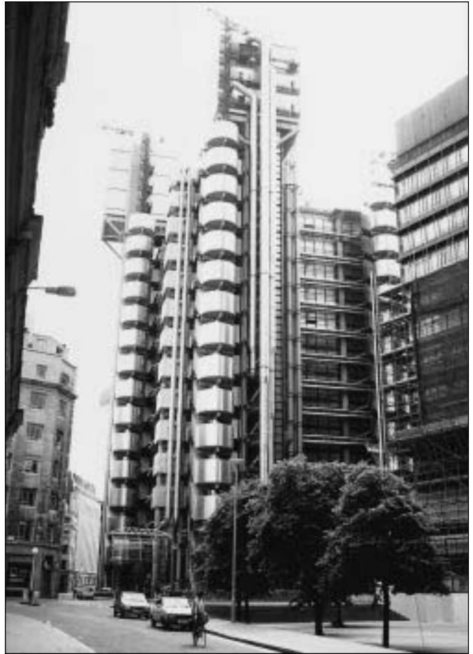
Fig. 7.9 Lloyd's headquarters building, London, UK, 1986; Richard Rogers and Partners, architects; Ove Arup & Partners, structural engineers. The building has a rectangular plan and six projecting service towers.
