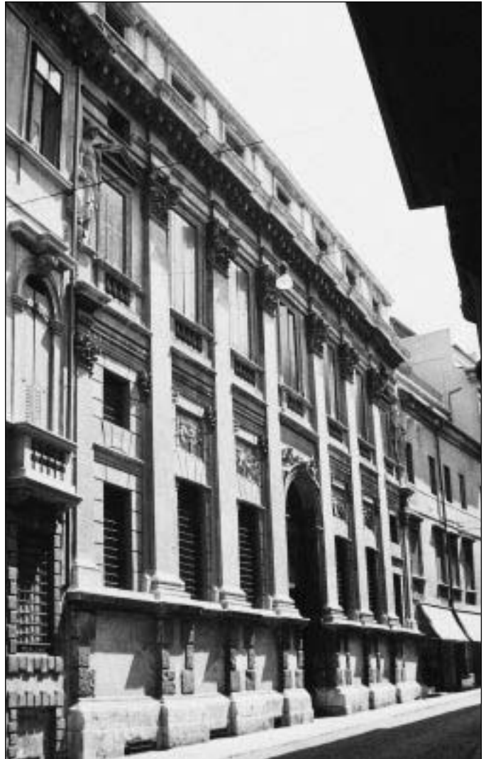
Fig. 7.2 The Palazzo Valmarana, Vicenza, by Andrea Palladio. The pilasters on this façade have their origins in a structural function but here form the outer skin of a structural wall. The architectural interest of the building does not lie in its structural make-up, however.
