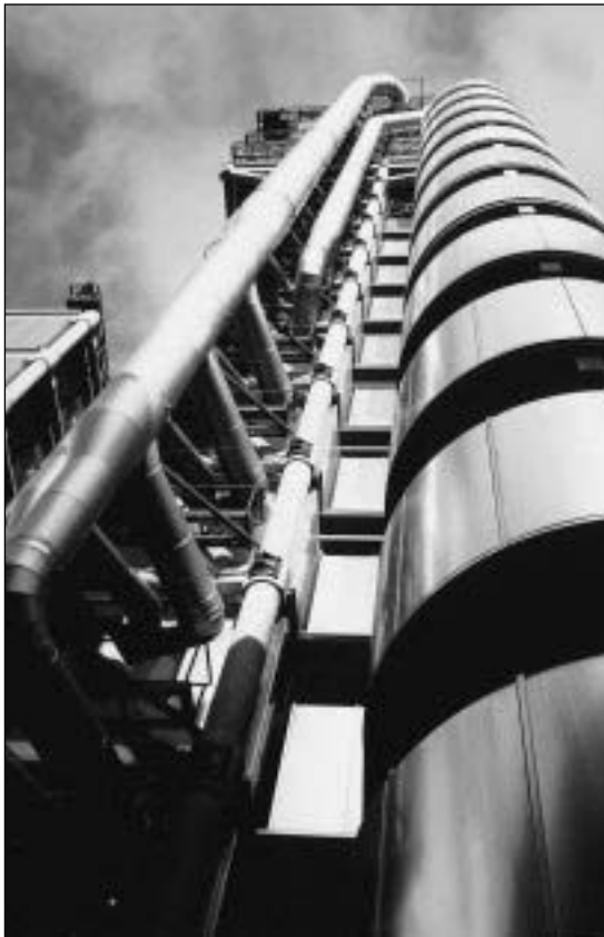
Fig. 7.11 Lloyds headquarters building, London, UK, 1986; Richard Rogers and Partners, architects; Ove Arup & Partners, structural engineers. The service towers which project from the rectangular plan are one of the most distinctive features of the building.
