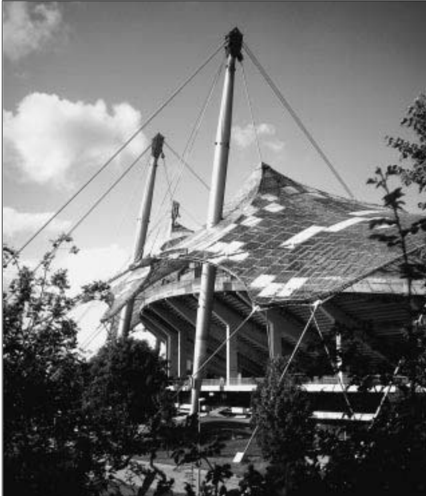
Fig. i Olympic Stadium, Munich, Germany, 1968–72; Behnisch & Partner, architects, with Frei Otto. In both the canopy and the raked seating most of what is seen is structural. (Photo: A. Macdonald)
