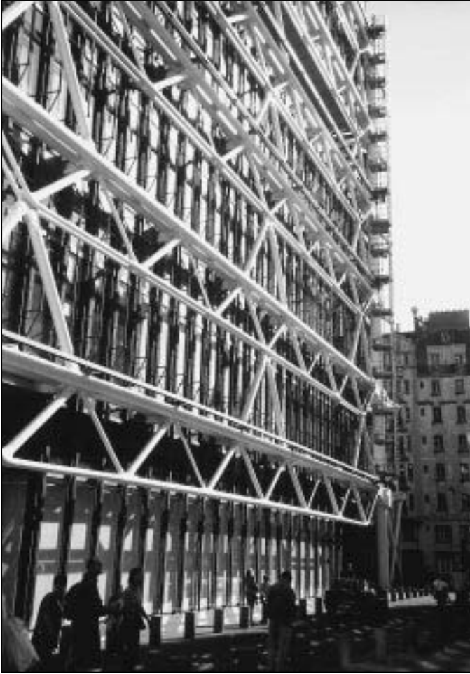
Fig. 1.10 Centre Pompidou, Paris, France, 1977; Piano & Rogers, architects; Ove Arup & Partners, structural engineers. The separation of structural and enclosing functions into distinct elements is obvious here. (Photo: A. Macdonald)
