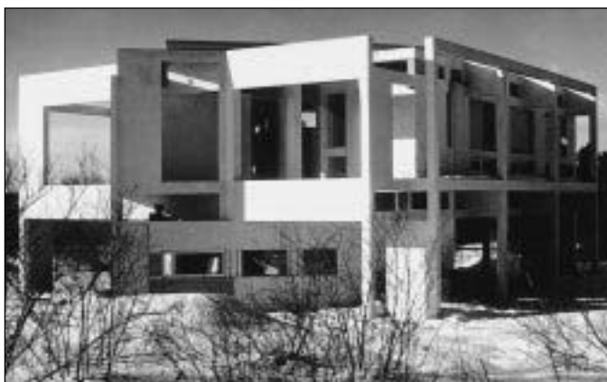
Fig. 5.18 Miller House, Connecticut, USA, 1970; Peter Eisenman, architect. Eisenman is one of a number of American architects, including Richard Meier (see Fig. 1.9), who have exploited the opportunities made possible by the continuous framework. This type of geometry, with its intersecting grids and contrasts of solid and void is only possible with a continuous structure.
