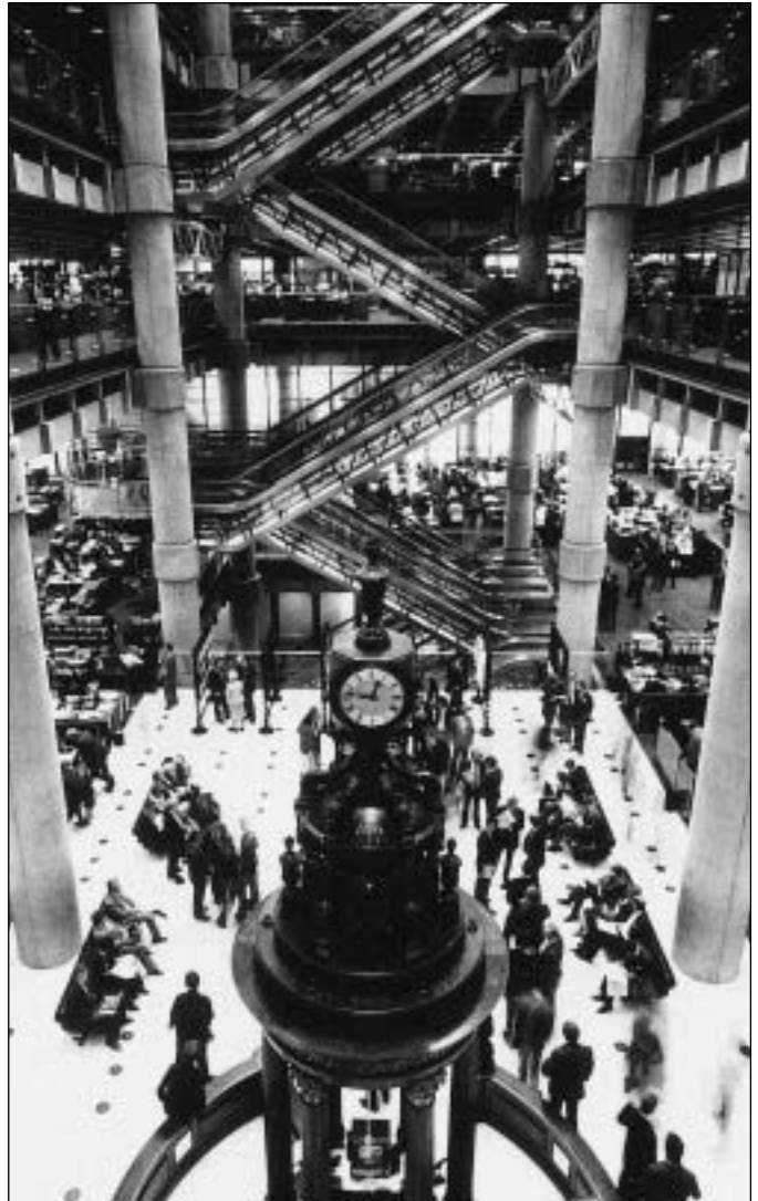
Fig. 7.12 Atrium, Lloyds headquarters building, London, UK, 1986; Richard Rogers and Partners, architects; Ove Arup & Partners, structural engineers. The columns are set outside the perimeter of the floor decks and connected to them through visually prominent pre-cast concrete brackets. The arrangement allows the structure to be easily 'read' but is far from ideal structurally. It introduces bending into the columns, which causes high concentrations of stress at the junctions.
