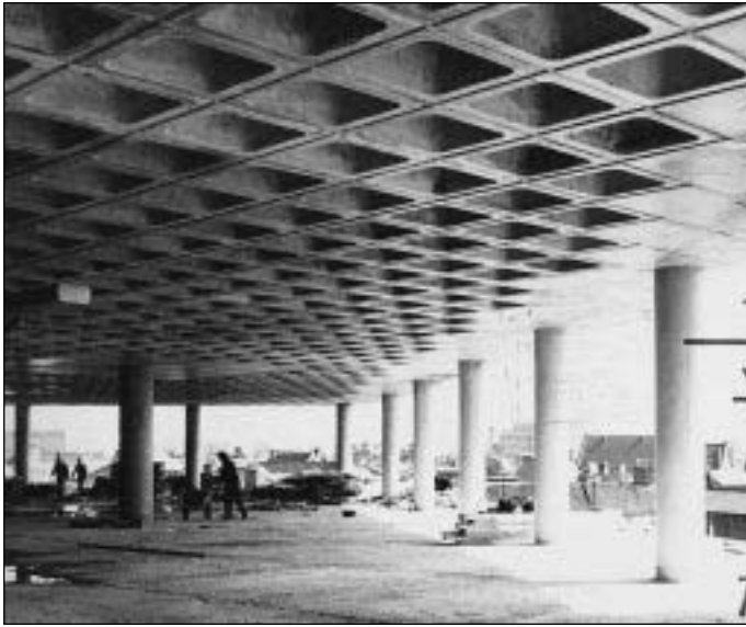
Fig. 5.19 Willis, Faber and Dumas office, Ipswich, UK, 1974; Foster Associates, architects; Anthony Hunt Associates, structural engineers. The coffered floor slab is a flat-slab structure with an 'improved' cross-section. (Photo: Pat Hunt)
