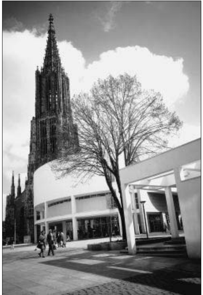
Fig. 1.9 Ulm Exhibition and Assembly Building, Germany, 1986–93; Richard Meier & Partners, architects. The mouldability of concrete and the structural continuity which is a feature of this material are exploited here to produce a complex juxtaposition of solid and void. (Photo: E. & F. McLachlan)
