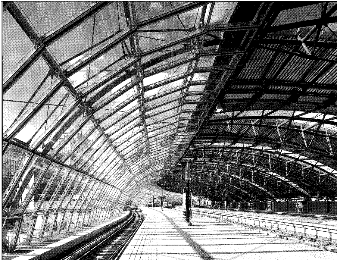
Fig. 7.17 International Rail Terminal, Waterloo Station, London, UK, 1992; Nicholas Grimshaw & Partners, architects; YRM Anthony Hunt Associates, structural engineers. This building is part of a continuing tradition of long-span structures for railway stations. The design contains a number of innovative features, most notably the use of tapering steel sub-elements. (Photo: J. Reid and J. Peck)
