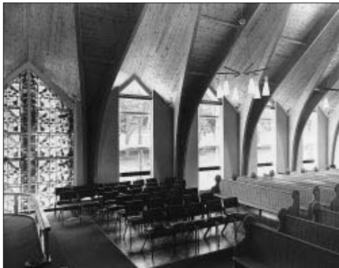
Fig. 3.4 Methodist church, Haverhill, Suffolk, UK; J. W. Alderton, architect. A series of laminated timber portal frames is used here to provide a vault-like interior. Timber is also used for secondary structural elements and interior lining. (Photo: S. Baynton)
