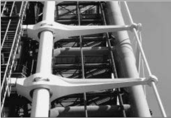
Fig. 7.7 Gerberette brackets, Centre Pompidou, Paris, France, 1978; Piano and Rogers, architects; Ove Arup & Partners, structural engineers. The floor girders are attached to the inner ends of these brackets, which pivot on hinge pins through the columns. The weights of the floors are counterbalanced by tie forces applied at the outer ends of the brackets. The arrangement sends 25% more force into the columns than would occur if the floor beams were attached to them directly. (Photo: A. Macdonald)
