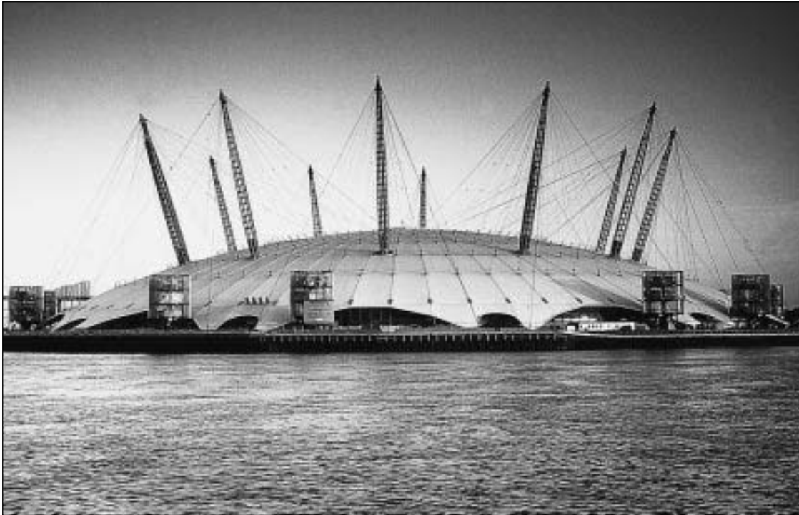
Fig. 7.19 Millennium Dome, London, UK, 1999; Richard Rogers and Partners, architects; Buro Happold, structural engineers. This is mast-supported, dome-shaped cable network with a diameter of 358 m. The use of a tensile form-active structure is fully justified for structures of this size.
