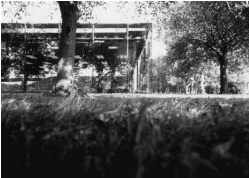
Fig. 7.38 IBM pilot head office, Cosham, UK, 1973; Foster Associates, architects; Anthony Hunt Associates, structural engineers. Intended as temporary accommodation, Foster and Hunt provided a stylish building for the same cost and within the same time-scale as those of a cluster of temporary buildings, which is what the client originally envisaged. The form adopted was to a large extent dictated by structural requirements. (Photo: Anthony Hunt Associates)
