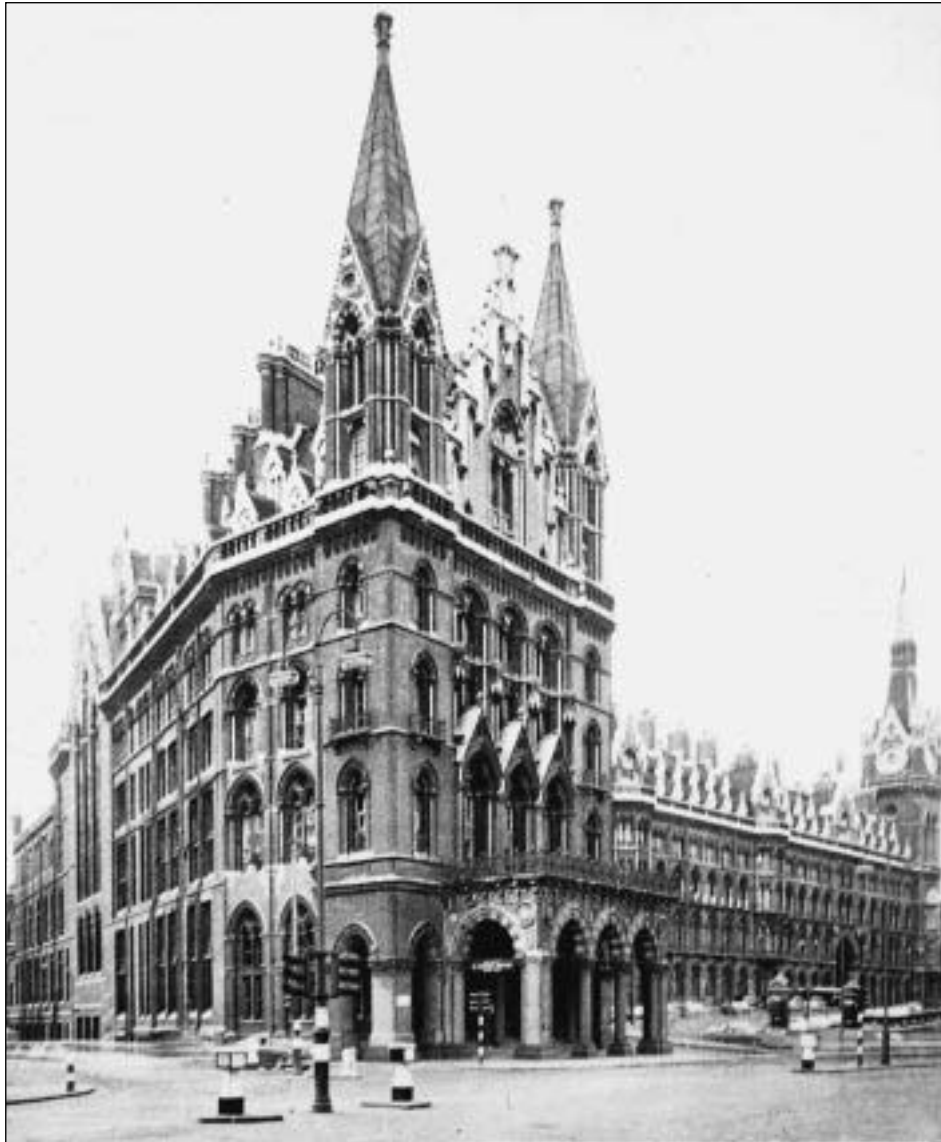
Fig. 7.52 Midland Hotel, at St Pancras Station, London, UK, 1871; G. Gilbert Scott, architect. The form of the train shed did not influence the architectural agenda at St Pancras.
