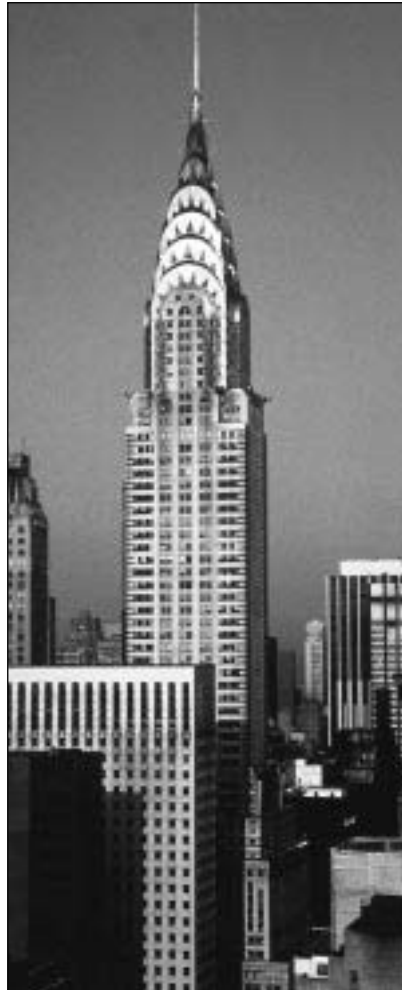
Fig. 7.35 Chrysler Building, New York, USA, 1930; William Van Allen, architect. Although the overall forms of Modernistic skyscrapers such as the Chrysler Building are determined by the steel frame structure the visual treatment is not. (Photo: Petra Hodgson)
