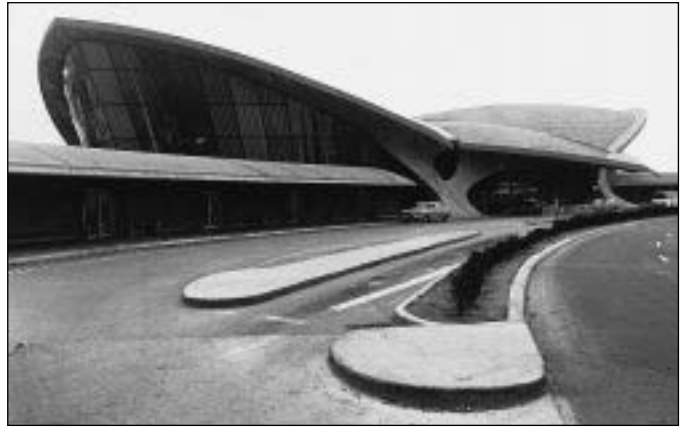
Fig. 7.45 TWA Terminal, Idlewild (now Kennedy) Airport, New York, USA, 1962; Eero Saarinen, architect; Amman and Whitney, structural engineers. The form here was far from ideal structurally and strengthening ribs of great thickness were required at locations of high internal force. The structure was therefore inefficient but construction was possible due to the relatively modest spans involved. (Photo: R. J. Mainstone)
