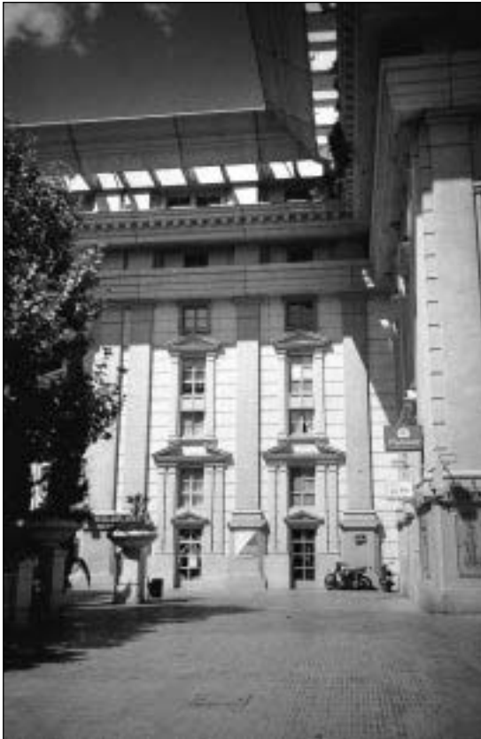
Fig. 1.8 Antigone, Montpellier, France, 1983; Ricardo Bofill, architect. This building is supported by a reinforced concrete framework. The exterior walls are a combination of in situ and pre-cast concrete. They carry their own weight but rely on the interior framework for lateral support. (Photo: A. Macdonald)
