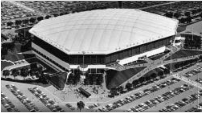
(a) Fig. 5.24 Barton Malow Silverdome. A very large span is achieved here with a cable-reinforced air-supported membrane, which is a tensile form-active structure.
