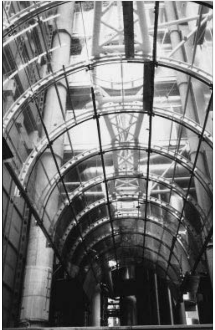
Fig. 7.5 Entrance canopy, Lloyds headquarters building, London, UK, 1986; Richard Rogers and Partners, architects; Ove Arup & Partners, structural engineers. The curved steel ribs with circular 'lightening' holes are reminiscent of structures found in the aerospace industry. (Photo: Colin McWilliam)
