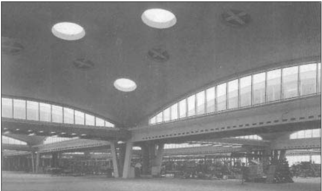
Fig. 5.25 Brynmawr Rubber Factory, Brynmawr, UK, 1952; Architects Co-Partnership, architects; Ove Arup & Partners, structural engineers. The principal enclosing elements here are compressive form-active, elliptical paraboloid shell roofs. (Photo: Architectural Review )
