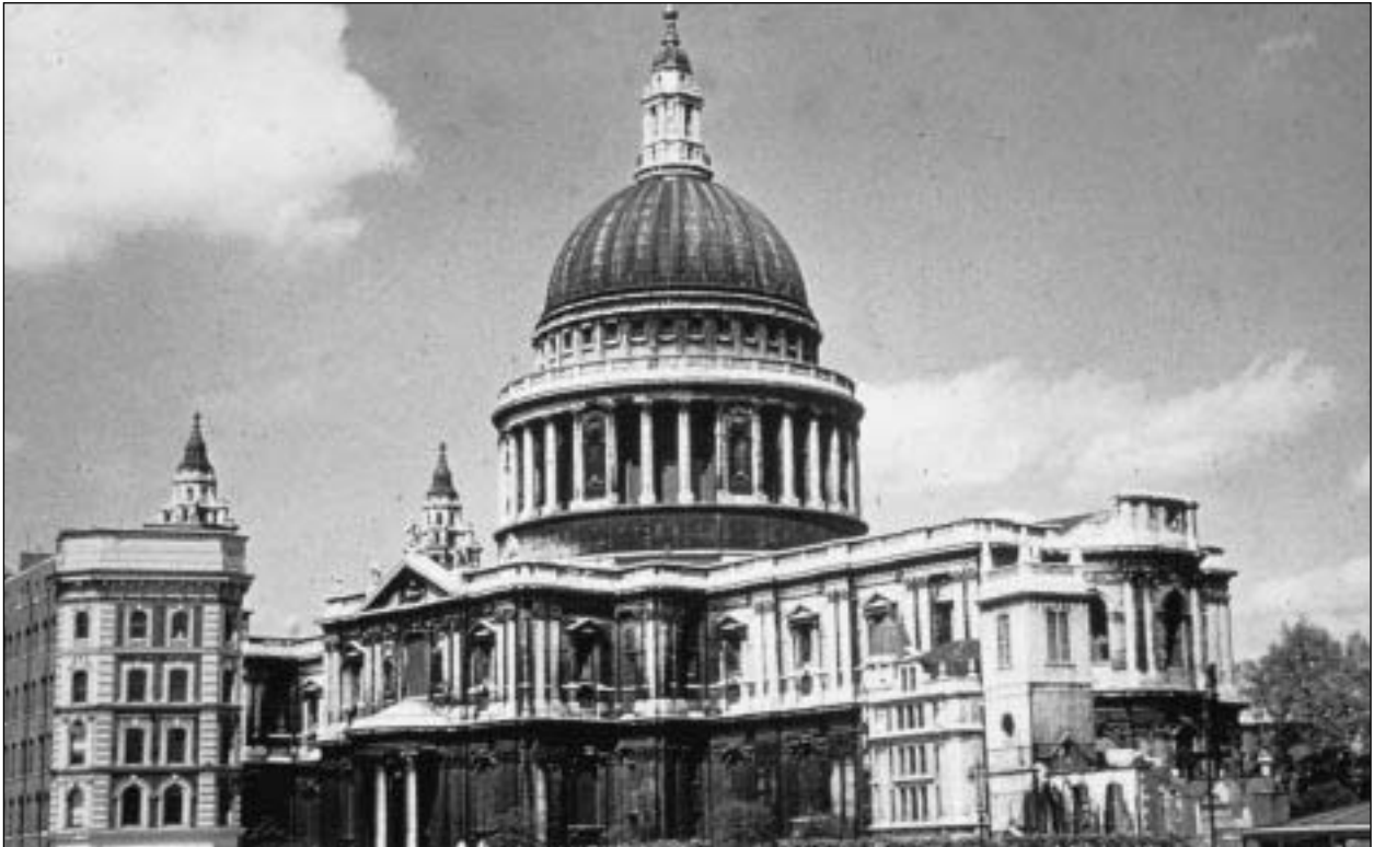
Fig. 7.48 St Paul's Cathedral, London, UK, 17th century; Sir Christopher Wren, architect. In treatment of both the dome and the exterior wall the structural arrangement is not reflected in the visual programme.
