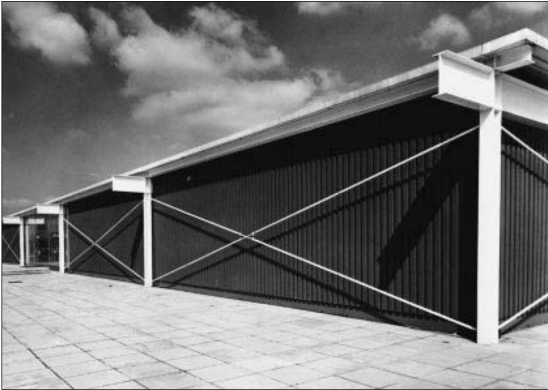
Fig. 7.4 Reliance Controls building, Swindon, UK, 1966; Team 4, architects; Tony Hunt, structural engineer. The exposed structure of the Reliance Controls building formed an important part of the visual vocabulary. It was modified in minor ways to improve its appearance. (Photo: Anthony Hunt Associates)
