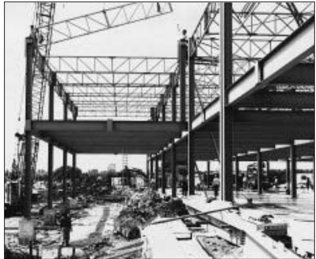
Fig. 5.13 'Improved' elements are used for all beams and columns in steel frames. In this case I-section beams are used for the floor structure and more efficient triangulated elements in the roof. The greater complexity and higher efficiency of the latter are justified by the lighter roof loading (see Section 6.2). (Photo: Pat Hunt)
